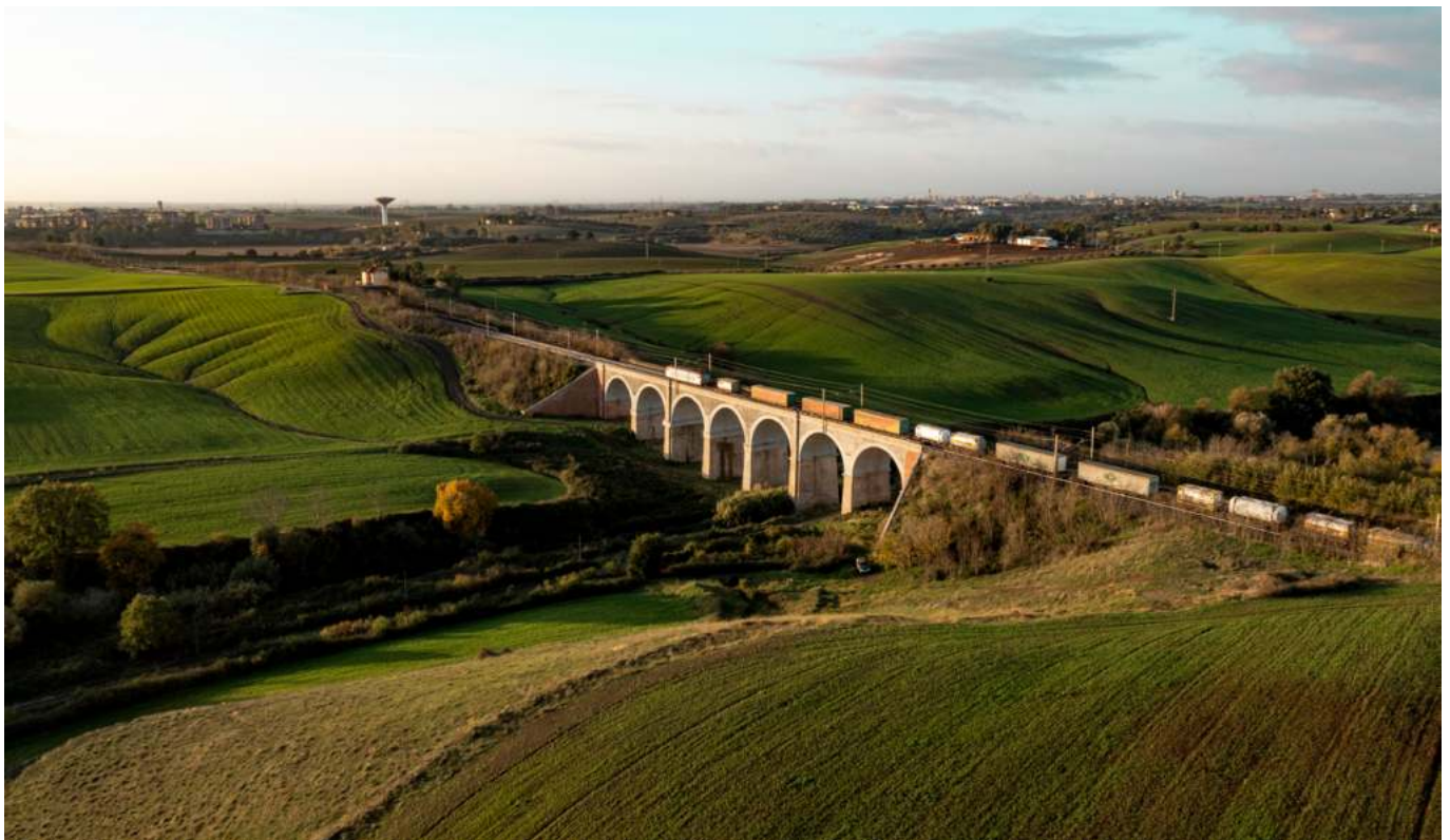
In-train communication realises real-time data transfer between the wagon and running locomotive in order to transmit safety and vehicle-related information Credit: Polo Logistica FS, free of charge
